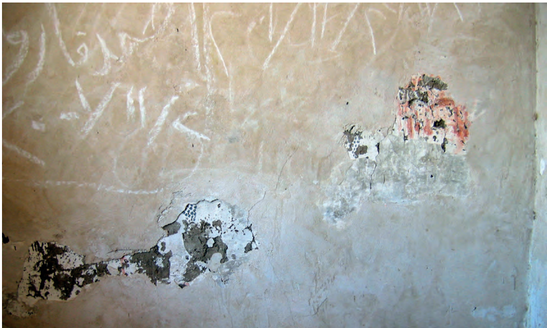
Abb. 10: Erdgeschoss, 1. Raum, Detail Westwand; 2005
