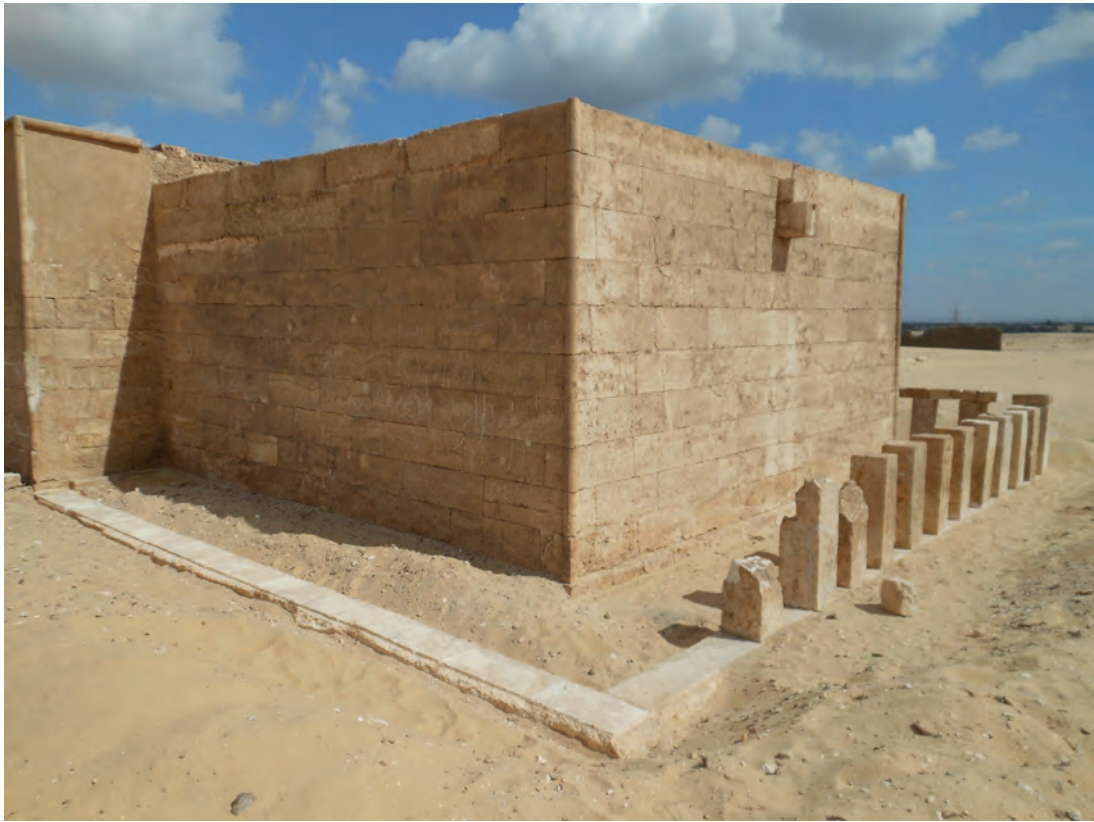
Fig. 3: The foundation of the balustrade in the west and south; 2015
