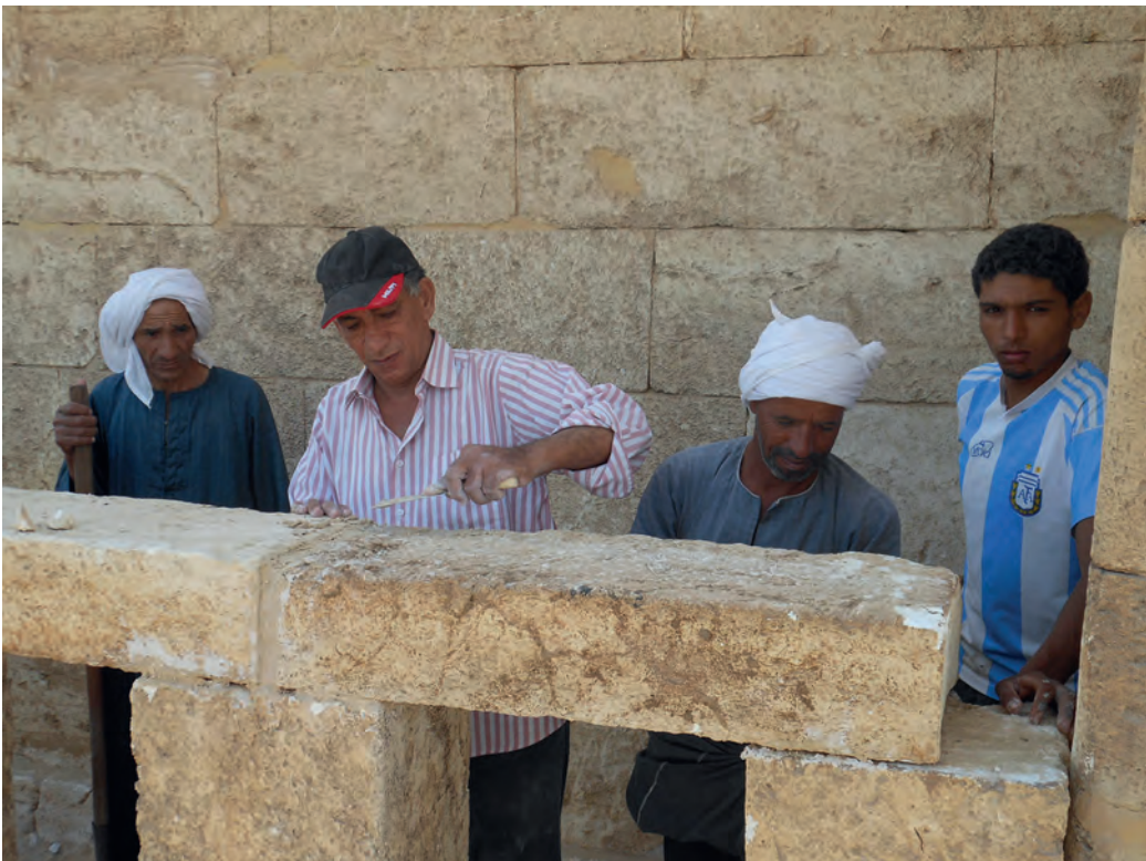
Fig. 14: Re-erection of balustrade with the help of lime mortar; 2015
