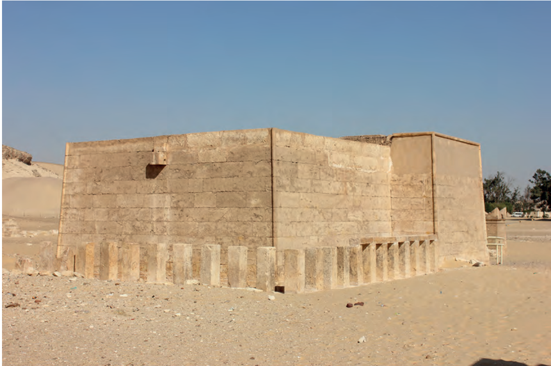
Fig. 1: The re-erected balustrade on the eastern and southern side of the tomb of Petosiris (GB 50); 2015
