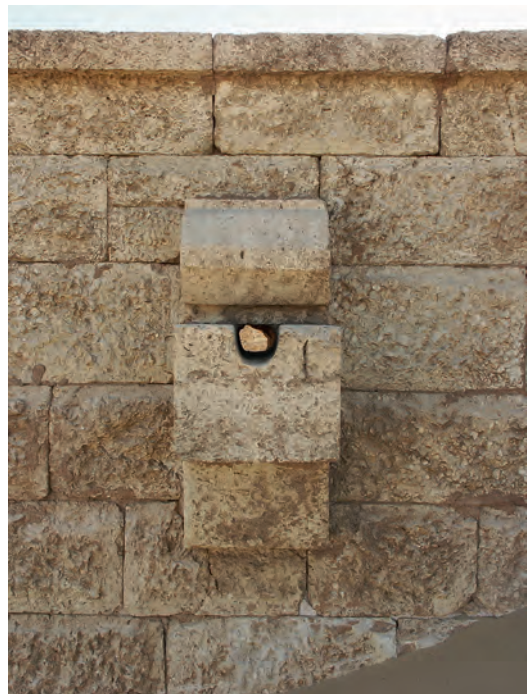
Abb. 9: Westwand, Wasserspeier; 2006
