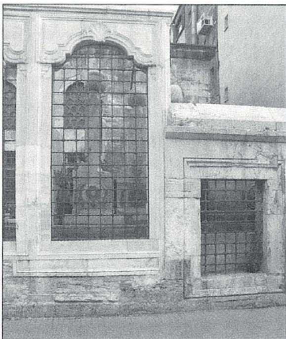
Fig. 74: Detail of the Koca Sinan hazire openings.
